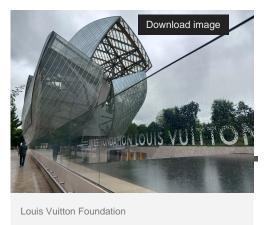
Louis Vuitton Foundation, designed by the renowned architect Frank Gehry, is a masterpiece of contemporary architecture. One of the key aspects in the construction of this iconic building is the use of duplex stainless steel, an alloy that combines properties of both austenitic and ferritic stainless steel.
