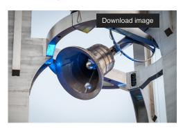
This sophisticated musical instrument, Ars Sonora, is made up of 63 bronze bells electrically connected to a keyboard so that each key is responsible for controlling the sound generated by each bell. It is supported by a metallic structure made of 5.2 tons of rectangular stainless steel tube with a hollow section.
