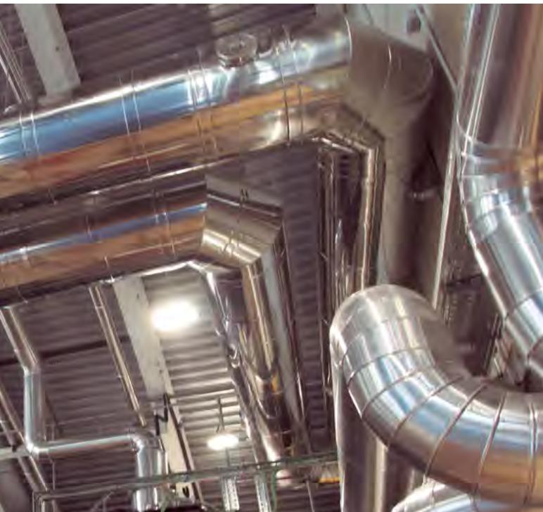
*The installation consists of 2 biomass boilers of 1.4 MW with modular chimney systems DW ECO 316 of 600 mm diameter made in AISI 316 stainless steel (60 m chimney in total); 2 gas boilers with 2.3 MW with additional heat exchanger also installed with the modular chimney system DW ECO 316 condensing (70 m of chimney in total); and a 200 kVA generator set with a chimney of approximately 20 m in DW-KL 50 exhaust system in diameter 150mm.*
