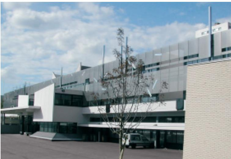
*In this school building stainless-steel grilles perform a dual function – as façade cladding and as solar shading for the classrooms behind.*
