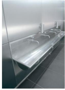
All the workings are concealed securely inside this unit, giving excellent protection against damage and vandalism.
