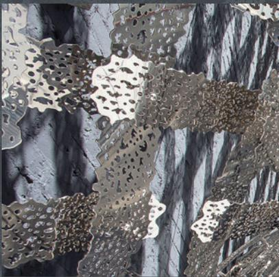
A complex structure and engineering feat, the “foliage” ribbons are laser-cut out of 11-gauge (3mm) 316L alloy (UNS S31603) stainless steel and polished with a #4 non-directional finish on the back and a #7 mirror finish on the front.
