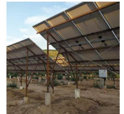
*Mounting structures consist of piles for ground mounting, legs, column, beams, rail and clamps, and other assembly fixtures.*
