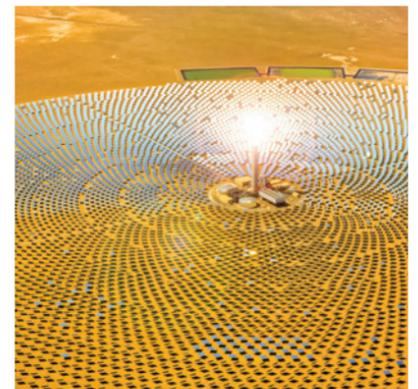
*Concentrated solar power (CSP) uses mirrors to reflect, concentrate and focus sunlight onto a receiver, which collects and transfers solar energy to a heat transfer fluid.*
