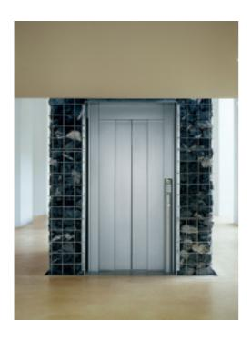
The cabin cladding of patterned, rolled stainless steel (2W) at the University of Vaduz blends well with the rubble masonry of the lift-shaft walls.
