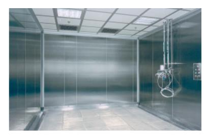
In this cleaning room in a pharmaceutical company, the wall cladding and the floor grating are made out of stainless steel (grade: 1.4301).
