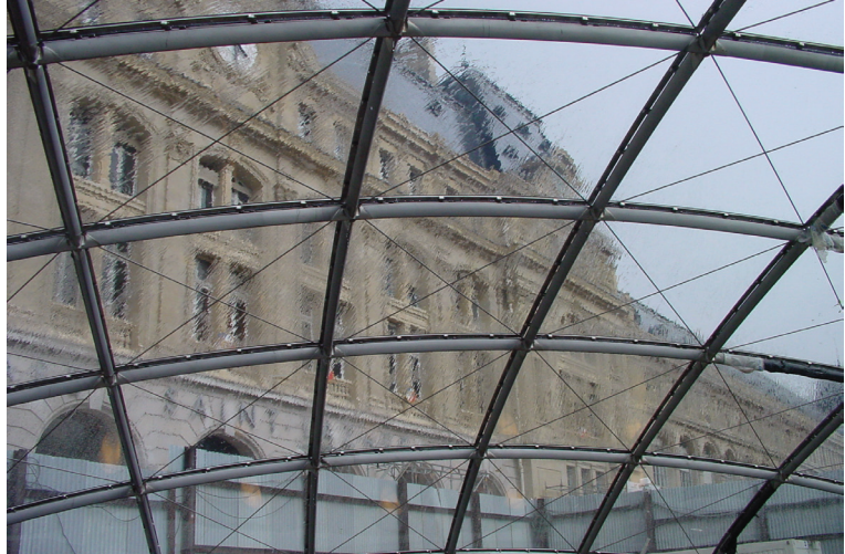
Photo 7: The glass-steel structure “La lentille de la cour de Rome” (The lens of the Rome yard) – Paris (F)
