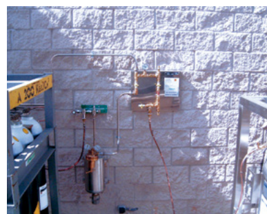
Starcyl panel and back up with simple manifold 1 bundle. COURTESY OF NIPPON GASES
