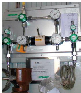
Stations of automatic change over. COURTESY OF NIPPON GASES
