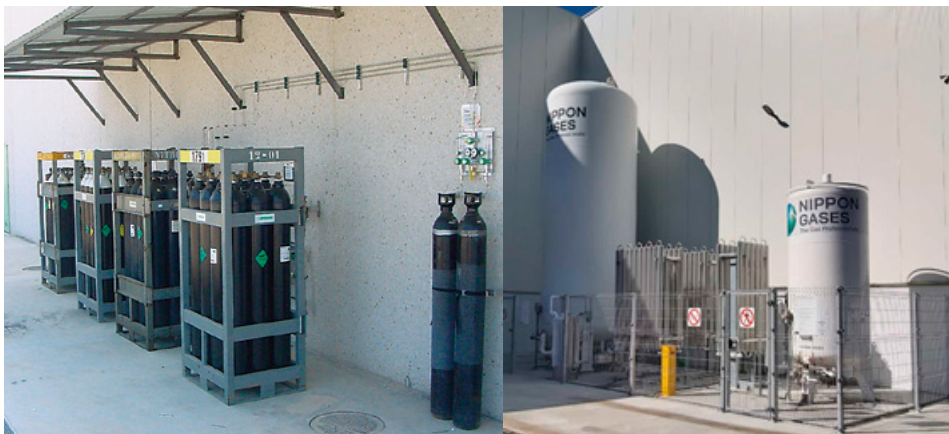
Fig. 121 - Supply of assist gas. COURTESY OF NIPPON GASES
