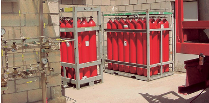
Fig. 109 - Supply of H_2 with installation of H_2 with semi-trailer with battery reserve 1+1 blocks. COURTESY OF NIPPON GASES
