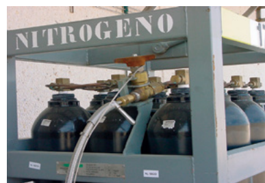
Double manifold 1+1 bundles of N COURTESY OF NIPPON GASES
