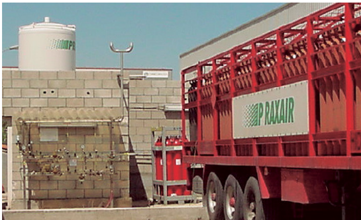
Fig. 110 - Complete facility to supply atmosphere H_2+N_2 o H_2+Ar . COURTESY OF NIPPON GASES
