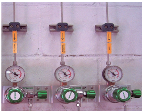
Fig. 119 - Double panels 1+1 cylinders and workstation of He-50; N 2 -50; CO 2 -48. COURTESY OF NIPPON GASES
