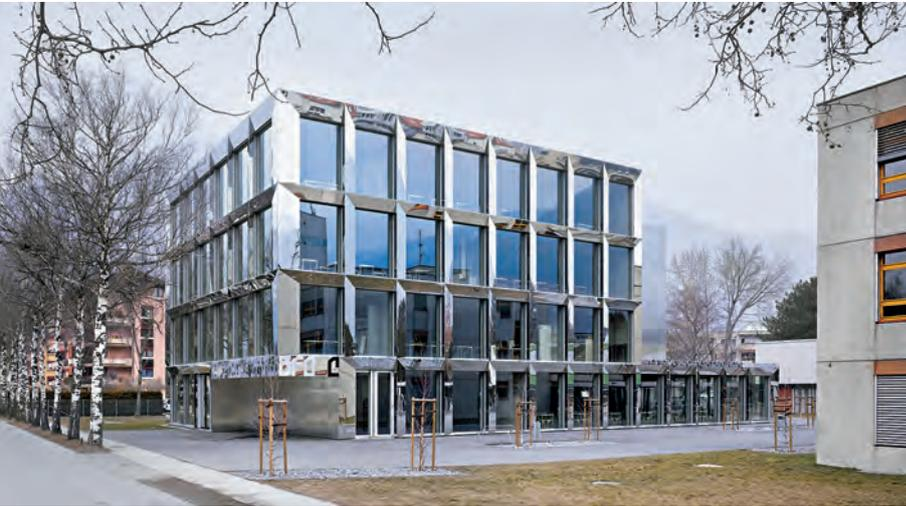
*Although conforming to the surrounding development in terms of volume, the new college building is quite different in looks, thanks to the mirror finish of its stainless steel cladding.*
