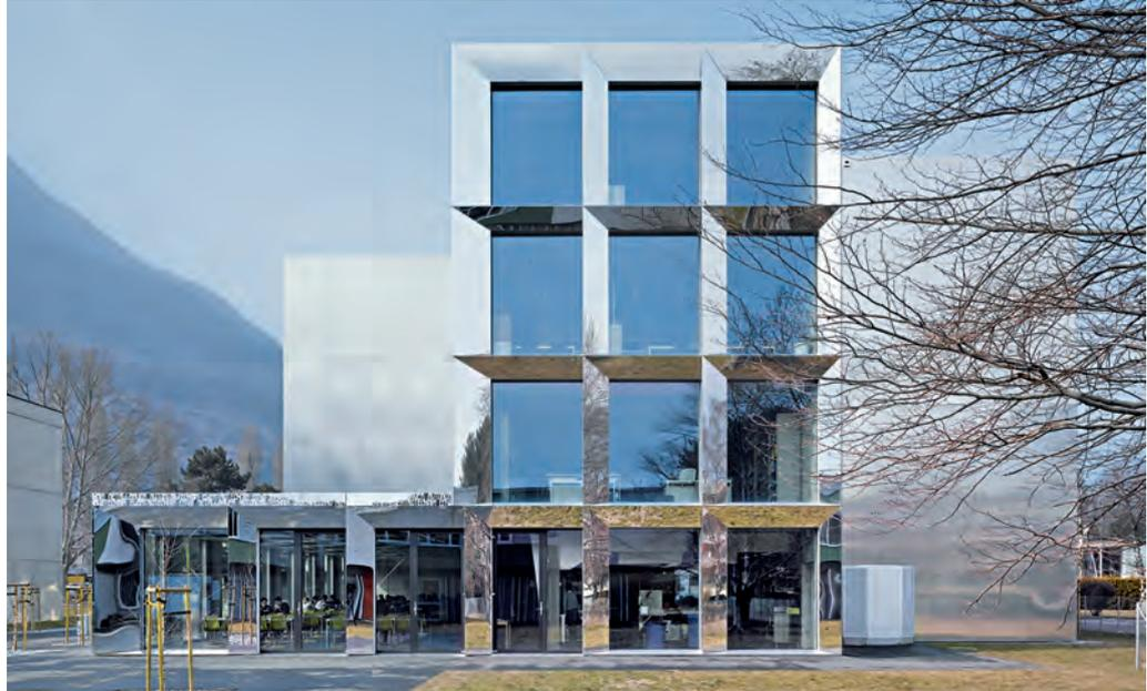
At each intersection in the cladding eight surfaces converge at different angles of inclination, a factor which made designing and constructing this detail a tricky task. The narrow space between the prefabricated load-bearing components of the reinforced concrete frame and the curtain wall is used to accommodate external louvre blinds to protect
