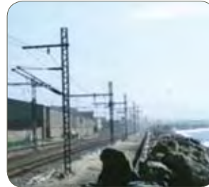
Grade 1.4003 (first major application in 1982, along seashore – 10m from surf, no corrosion), S. Africa
