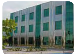
Partially 444 building cladding, Brazil.
