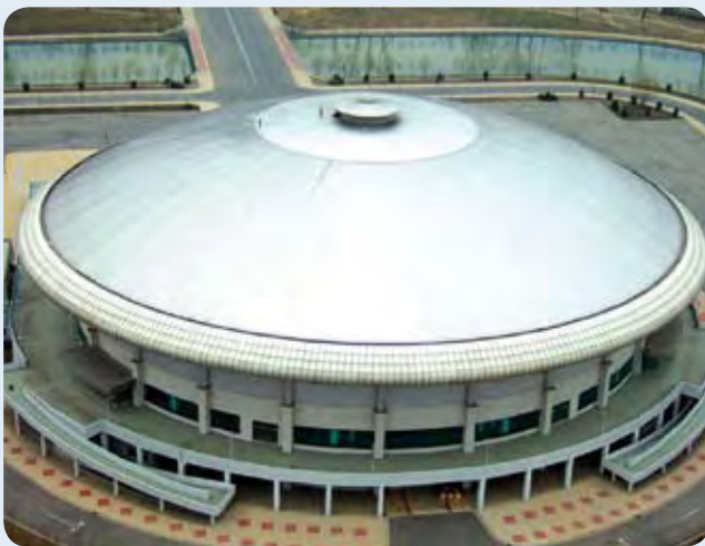
Gymnasium roof, in grade 445, S. Korea.
