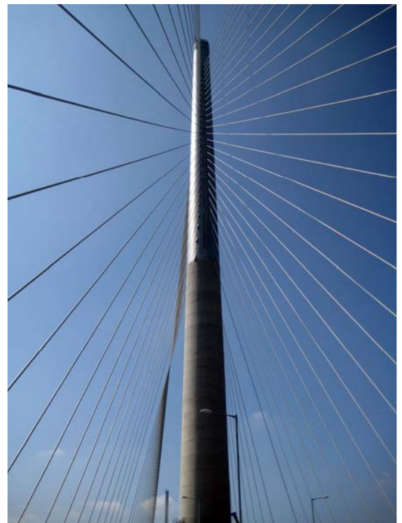
Figure 2: Mono tower and stay cables
