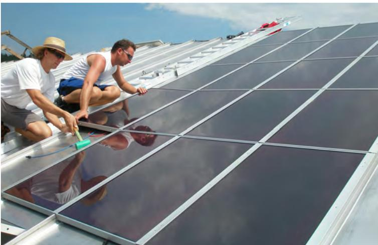
*The solar panels were fitted flush with the roof surface, between the stainless steel standing seams.*
