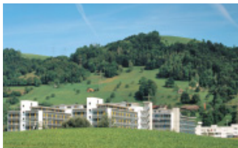
D4 Business Center, Lucerne, Switzerland Client: SUVA, Lucerne, Switzerland Architects: Fischer Architekten, Zürich, Switzerland Photo: Marsch & Company, Hamburg, Germany
