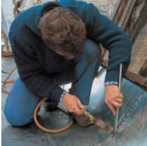
*Stainless steel is easy to solder if suitable flux and solder are used.*
