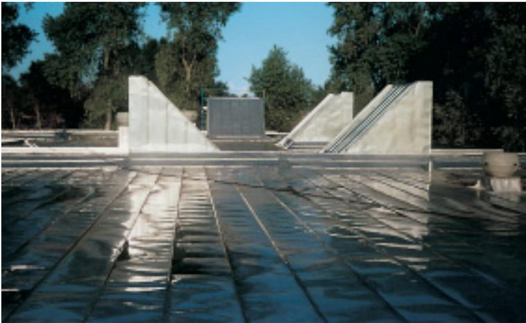
*A standard 2B mill finish offers a particularly cost-effective solution for flat roofs.*
