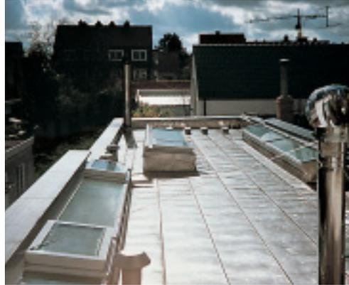
*Welded stainless steel is typically used on flat roofs with little or no slope for which no other metallic solution is appropriate.*
