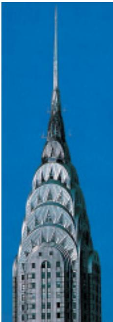
*Although it has only been cleaned once, the stainless steel roof of the Chrysler Building is still in excellent condition after more than 70 years.*
