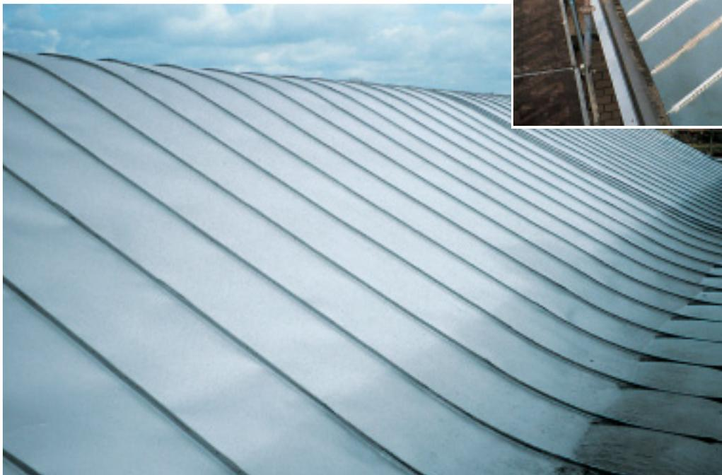
*Welded roofs can be used on most roof geometries.*
