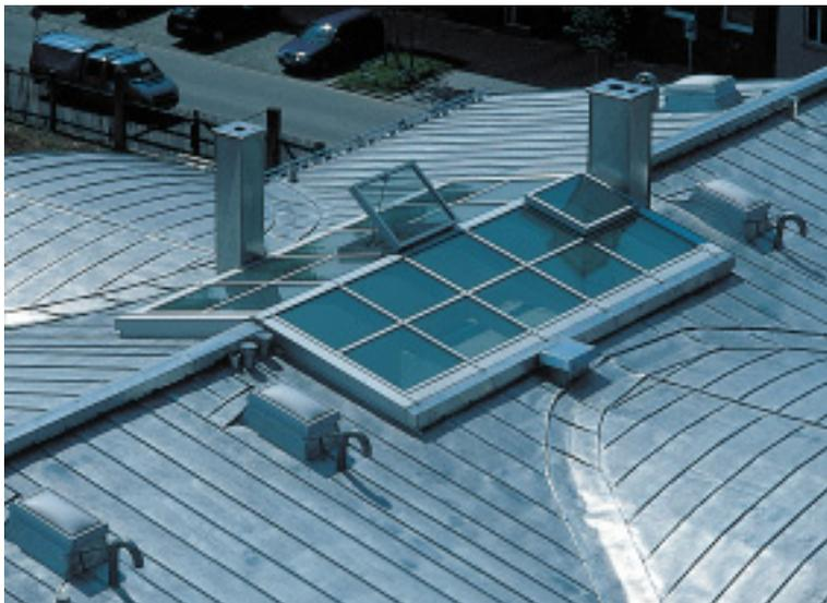
*Standing seam roofing is suitable for pitched and curved roofs.*
