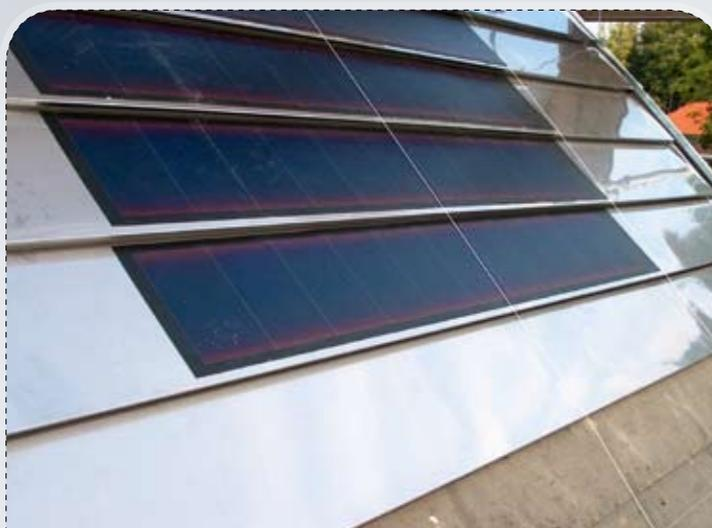
FIGURE 4: Detailed view of the stainless steel tilted roof in Stralsund. Active photovoltaic sections (centre) can easily be combined with non-active ones (right and left).
