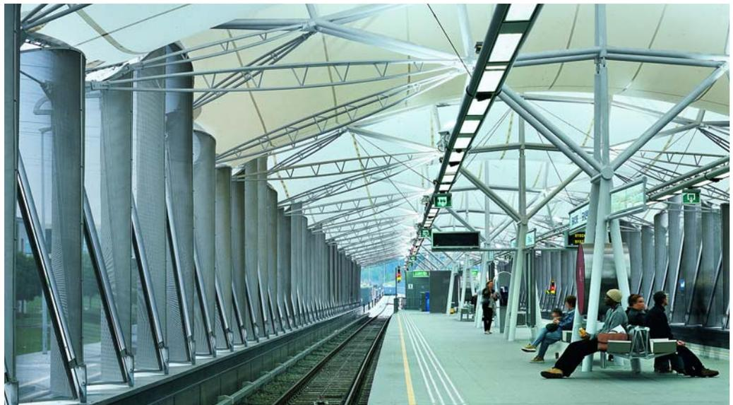
*The façade panels are of stainless-steel mesh (grade EN 1.4404) with an open area of 27%.*
