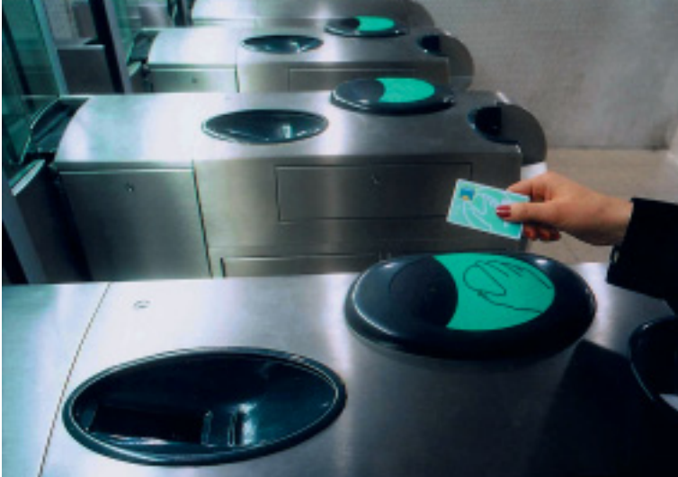
Line 14 makes use of a new stainless steel clad ticket dating system.
