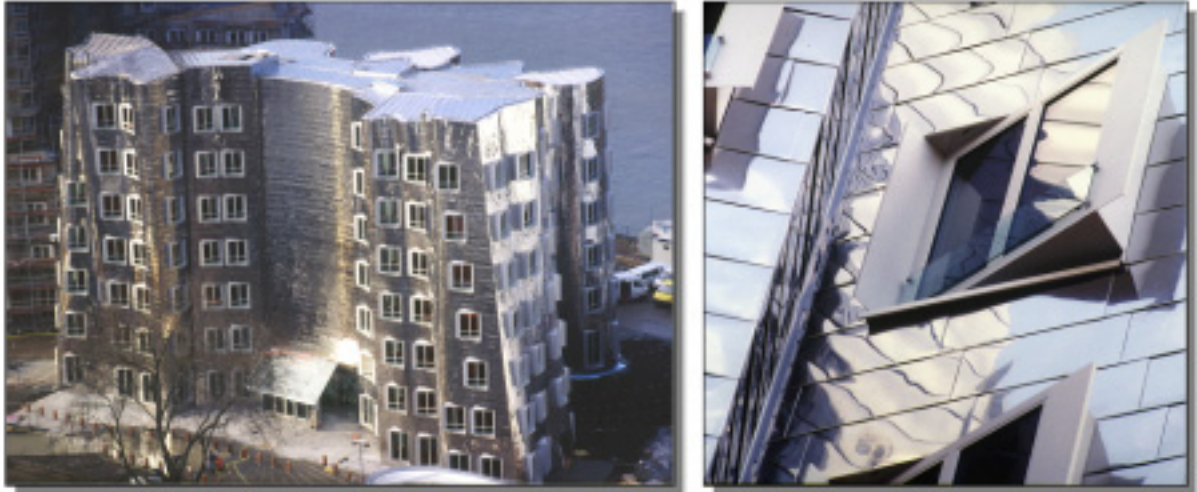
Facade worked in bright annealed stainless steel, Architect: Frank Gehry, USA Grade 1.4401 in 0.5 mm thickness.
