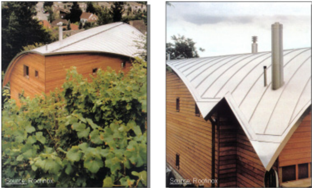
Stainless Steel as roofing material for domestic architecture. Grade 1.4301 (AISI 304) with matt-rolled surface, thickness 0.5 mm
