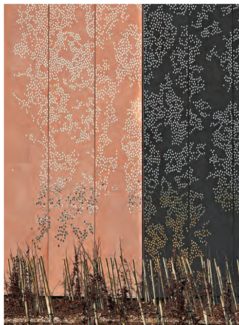
The pattern, which extends over all the facades, gradually disperses at the base of the building to create a transition from the earth-coloured concrete to the ground.
