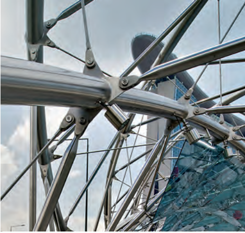
Compression and tension bars connect the tubular steel of the spirals.
