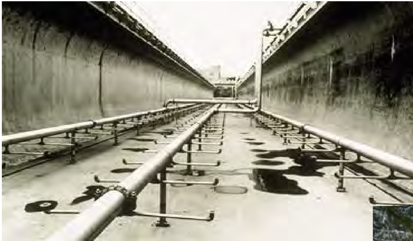
304 stainless steel piping after cleaning out basin, USA
