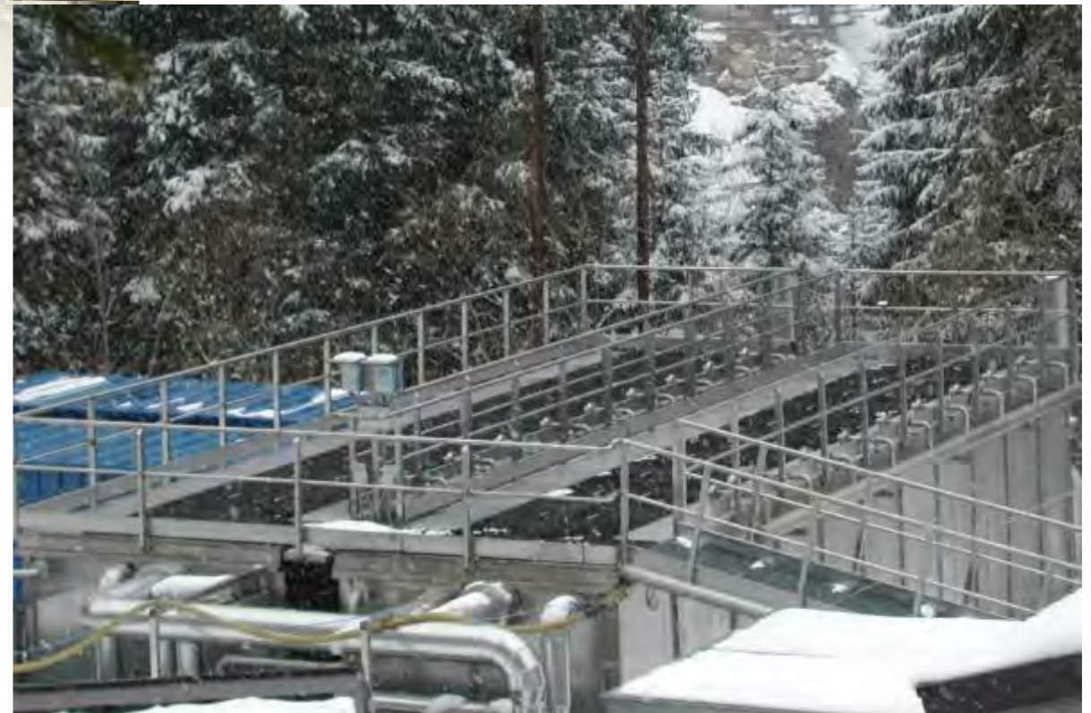
Two stainless steel containers with aeration tanks.
