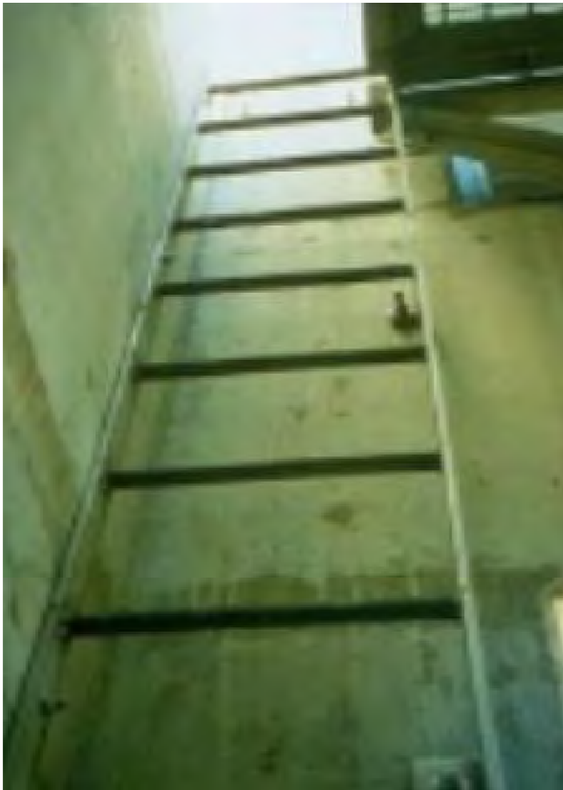
Ladders and fixings
