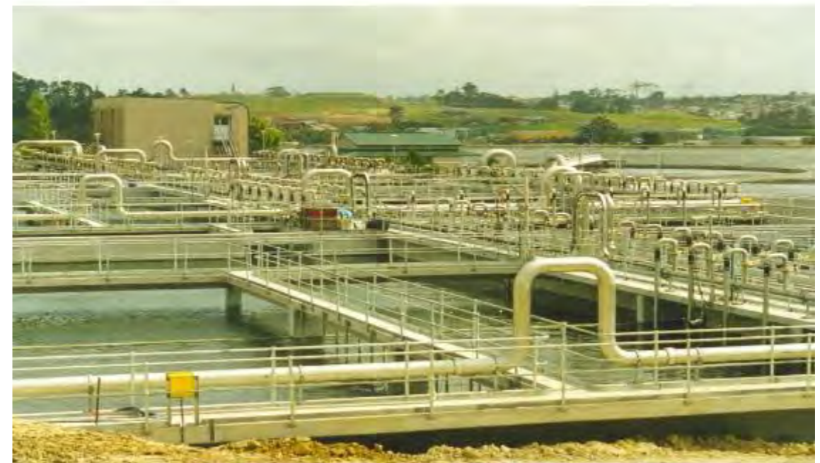
North Shore Waste Water Treatment Plant Auckland, New Zealand
