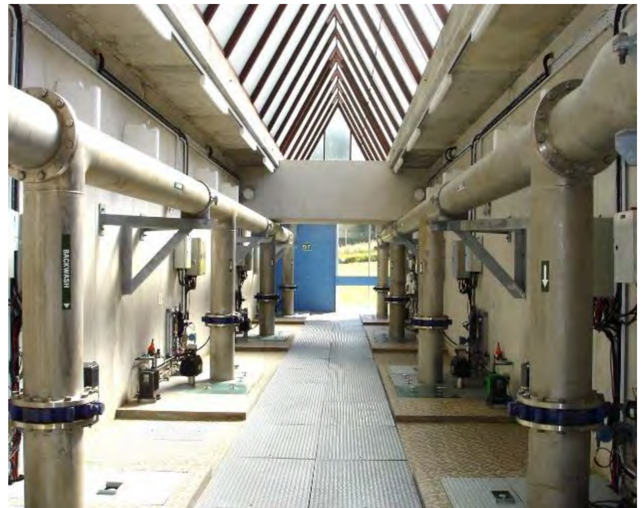
Piping gallery in water treatment plant, New Zealand
