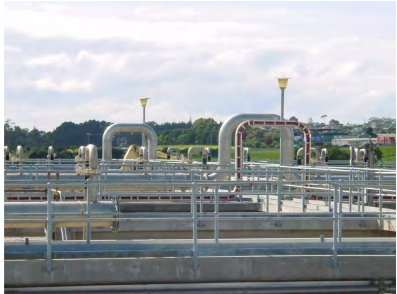
Duplex 2205 Biogas transfer piping at waste water treatment plant in New Zealand
