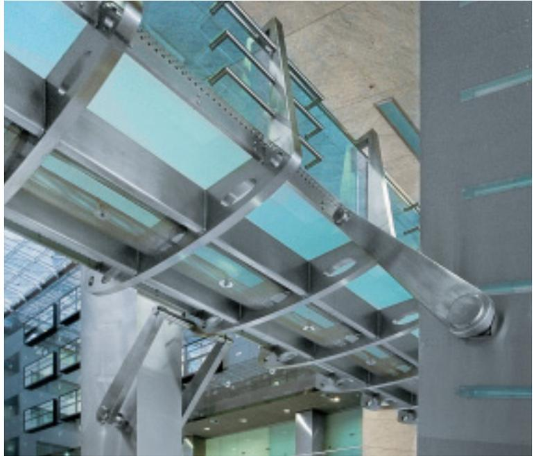
*At the mid-point of the walkway loads are directed down into the stainless-steel-clad columns.*
