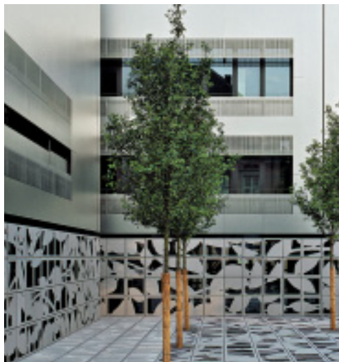
The electrically operated sun screens close smoothly to form a seamless stainless steel skin.
