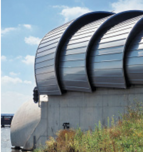
A range of alloys are available to meet the corrosion-resistance requirements of differing locations – the example here is of a coastal environment.
