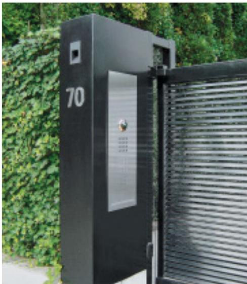
*The doorbell, intercom and house number are integrated in this entrance situation in a very neat and understated way. Stainless steel is particularly well suited for outdoor use because of its high corrosion-resistance and long service-life.*
