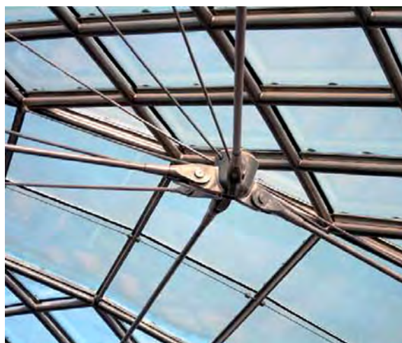
Figure 2: View of cast stainless steel joint with reflective glass
