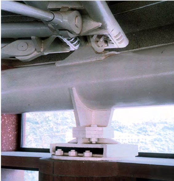
Figure 7: Support system for the VIP dome
