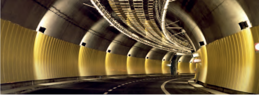
In corrosion-resistant tunnel liners, coil-coated stainless steel is used to avoid glare. Photo: ThyssenKrupp Acciai Speciali Terni, Terni (I)
