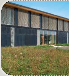
FIGURE 5: South facade with unglazed stainless steel solar collectors for floor heating and hot water. The connections between the absorber elements and the distribution pipes for the heat-transfer fluid are visible.
