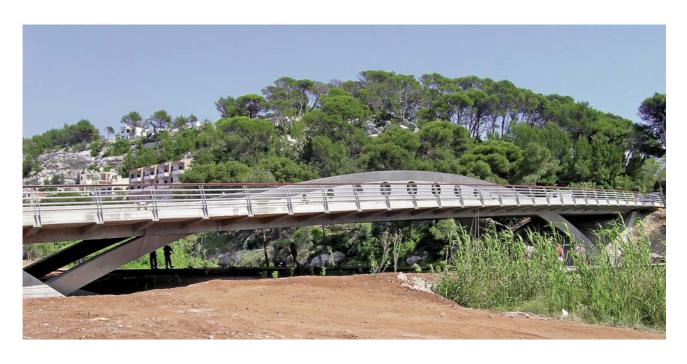
The inclined struts between the outer ends of the arches and the longitudinal beams take up the horizontal forces in the arches, thereby relieving pressure on the foundations.
