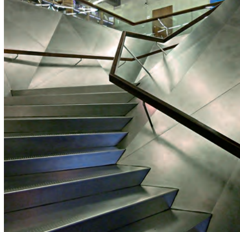
The dramatic spiral staircase leading to the lobby is clad entirely with sandwich panels surfaced with stainless steel.
