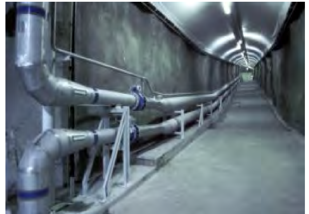
Lake Como Potable Water Plant, Italy
