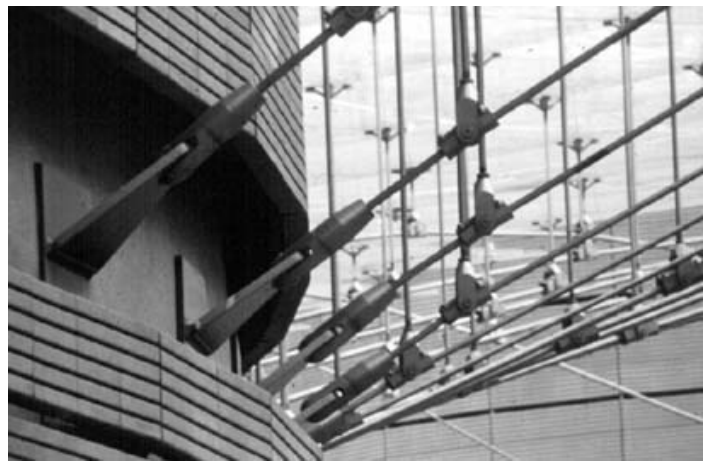
Anchoring and supporting elements of the tensile structure
