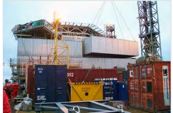
Figure 9: Installation of an accommodation module
