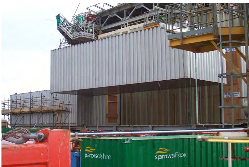
Figure 2: Installation of final module aboard the Armada Platform
