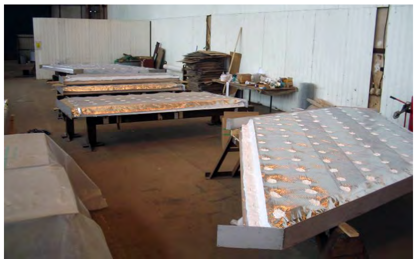
Figure 7: Insulation placed inside the wall panels
