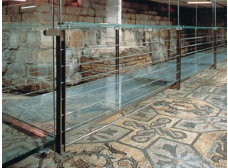
*Vertical glass panels on the corners, and horizontal tensioning bars counteract any oscillation tendencies in the walkway.*
