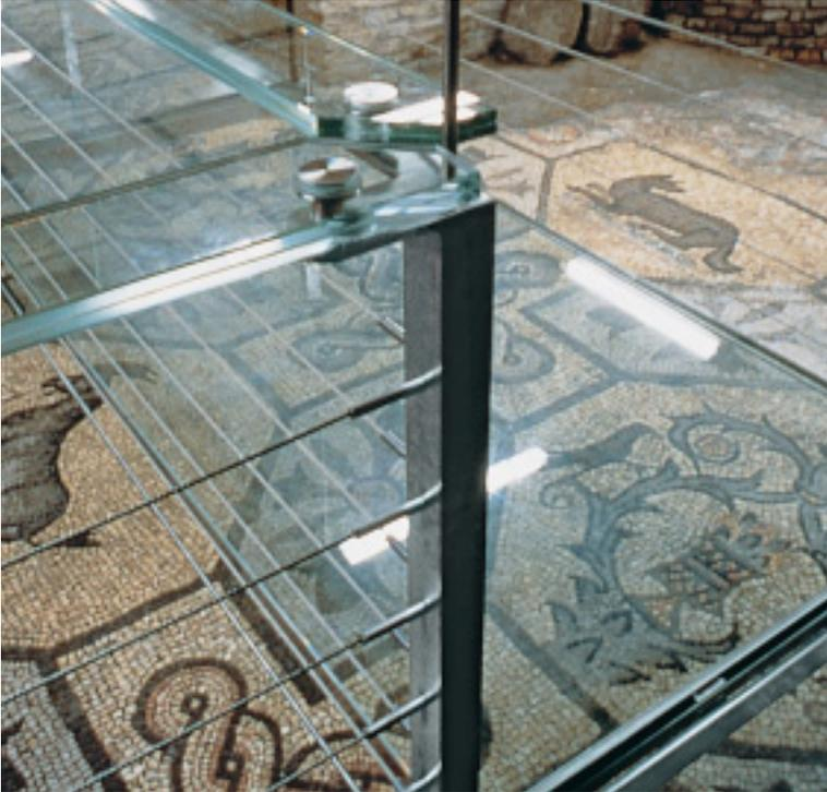
*The handrails, too, are of glass, so as not to impede the view of the mosaic floor.*
