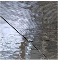
Some of the stainless steel panels on the ceiling are perforated with a 16 % open area and backed with acoustic fleece.
