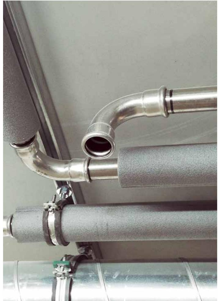
made out of ferritic stainless steel AISI 444- EN 1.4521, and especially its recognition by DVGW for sanitary water applications, has allowed to offer customers a very good alternative to austenitic steels with good value for
