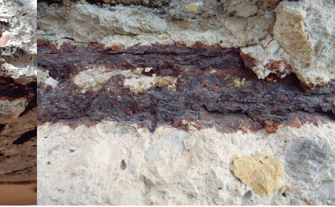
Figura 6: Oxidation remains in concrete
