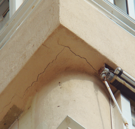
Figure 1: Fissures on the lower face of the slab front
