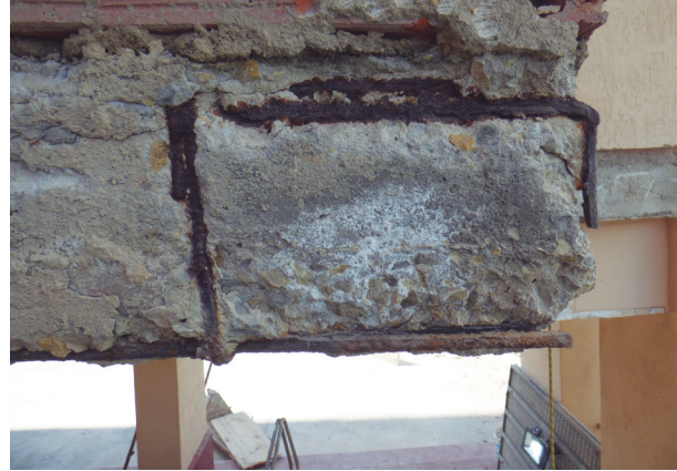
Figure 4: Slab front affected by oxidation
