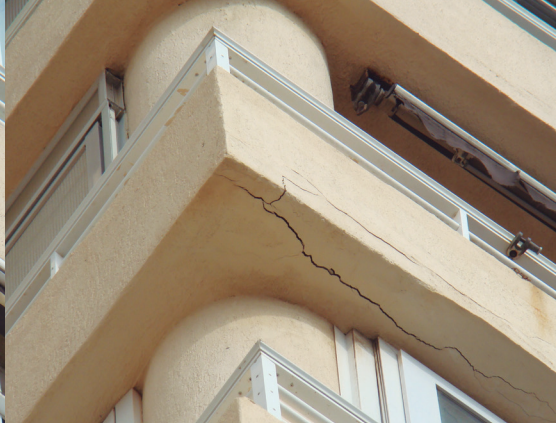
Figure 2: Fissures on the lower face of the slab front
