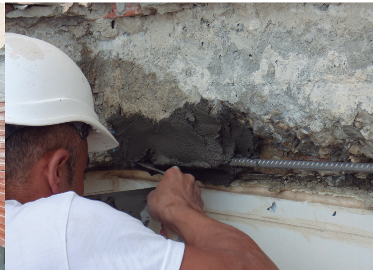
Figure 8: Retaking and regeneration of volume after placement of stainless steel rebar
