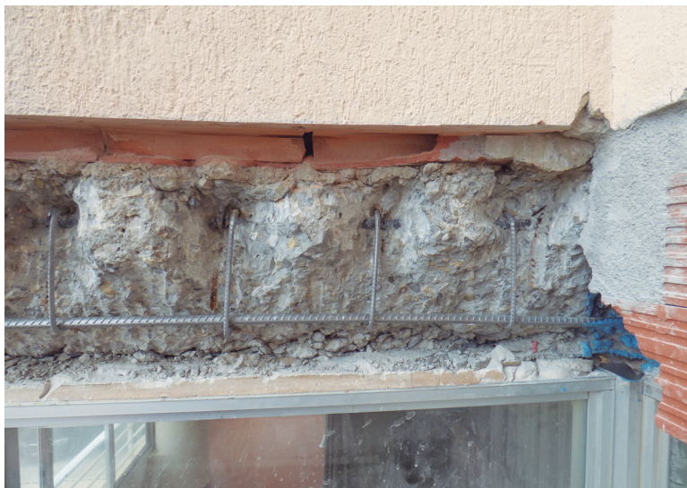
Figure 7: Placing of stainless steel reinforcement
