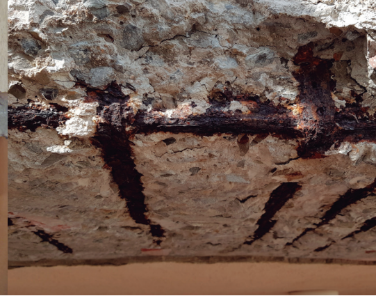
Figure 5: State of the reinforcements after coating removal
