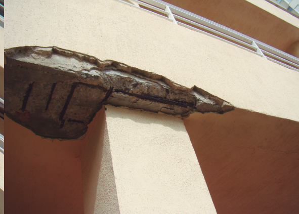
Figure 3: Detail of concrete spalling
