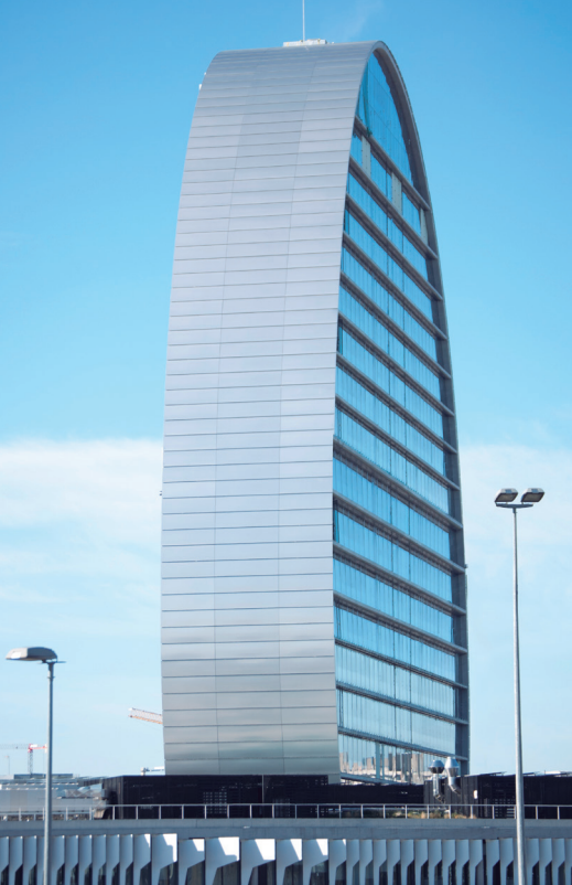
BBVA headquarters in Madrid. Stainless steel skin attached to each panel with 3M VHB™ tape (year 2015)
