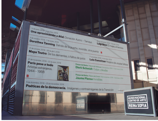
The Reina Sofia Museum, Madrid. Stainless steel plate glued to stainless steel plate with epoxy adhesive 3M™ Scotch-Weld 7260 B/A (year 2004)
