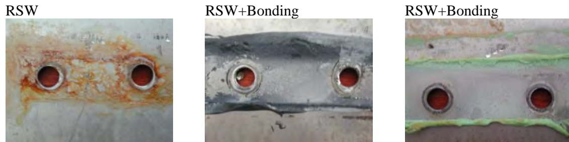
Figure 7. RSW not protected with rust formation, and RSW which are protected by the bonding after salt spray test
