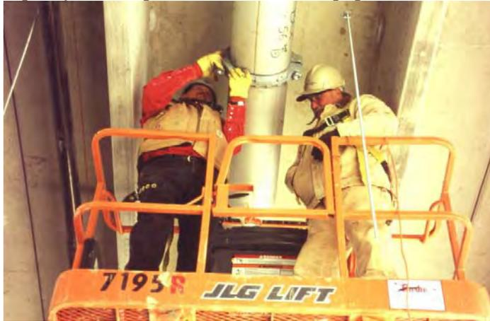
Figure 1. Installation of 300 mm drinking water piping in a sports stadium in Detroit, USA.
