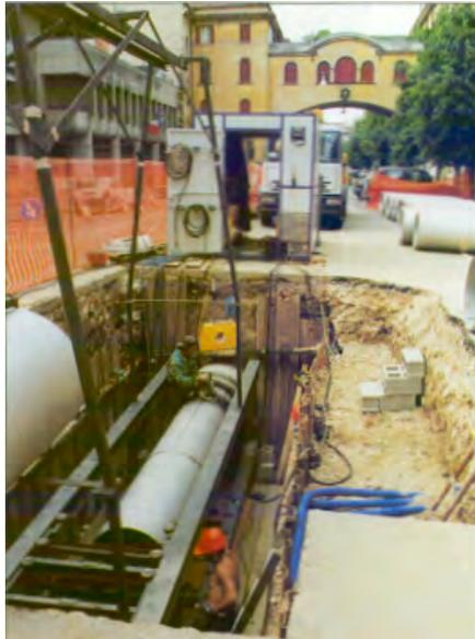
Figure 2. Trenchless relining of a water main in a busy street in Padua, Italy
