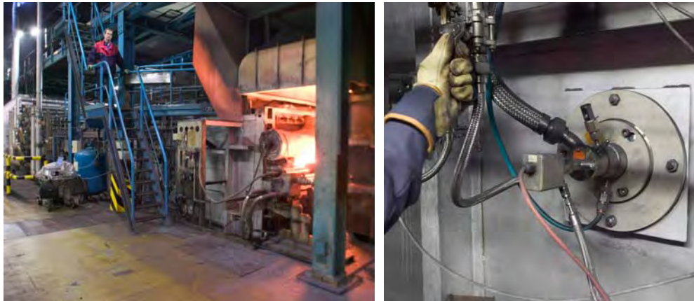
Figure 7. Flameless oxyfuel burner installation at Outokumpu, Nyby (fuel: oil).
