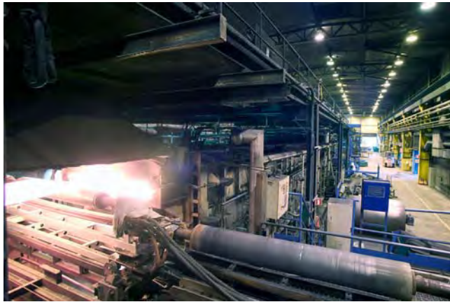
Figure 8. Flameless oxyfuel burner installation at Outokumpu, Avesta Works (fuel: oil).
