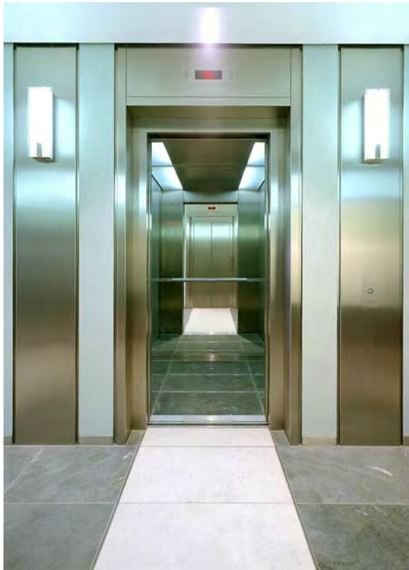
Figure 5 (above). Grade 1.4016 with a rolled-on satin finish applied in lift construction (Source: ThyssenKrupp Stainless)
