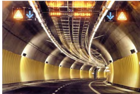
Figure 6 (above). Colour-coated stainless steel used as tunnel liner, to avoid reflections (Source: ThyssenKrupp Acciai Speciali Terni)
