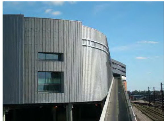
Figure 7 (above). Stainless steel roofing material used as cladding in the building envelope (Source: ArcelorMittal Stainless Europe)
