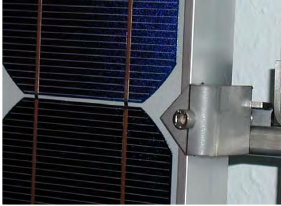
Figure 11. Fasteners made of grade 1.4362 Duplex stainless steel (Source: Modersohn)
