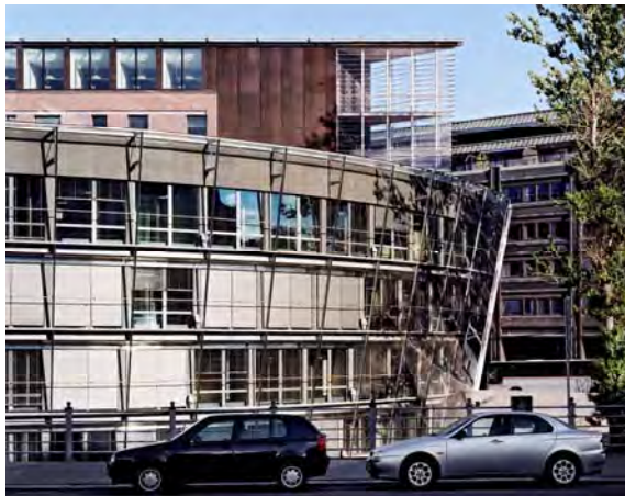
Figure 13. Glazed facade involving square hollow sections of stainless steel grade 1.4571 in the cold-worked condition CP350 (Source: Helin & Co Architects / M. Perlmutter)
