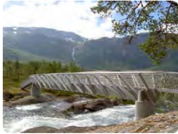
Figure 12. Bridge structure in grade 1.4162 Duplex stainless steel (Source: Outokumpu)
